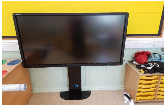
Before and after of the installed interactive boards.
